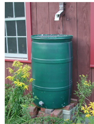
Rain Barrels conserve water by catching water from your rooftop for later use in your garden and flower beds.
