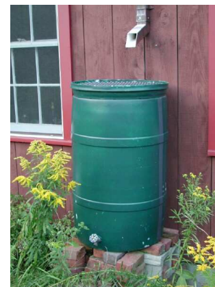
Rain Barrels conserve water by catching water from your rooftop for later use in your garden and flower beds.
