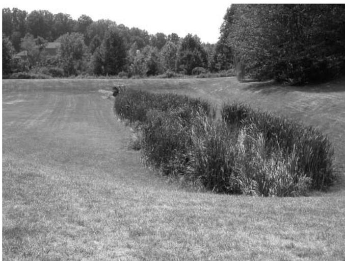
Biofiltration swales can be very effective in removing Total Suspended Solids (TSS) and adsorbed metals, although they are less effective in removing nutrients. While swales are not thought to be capable of quantity management, designs incorporating check dams can provide control of peak flows.
