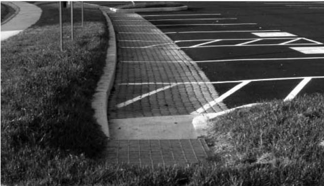
Porous pavement contains less fine aggregate in the mix to allow water to flow through the pavement to the stone reservoir below where runoff will be held until it is able to infiltrate into the existing soil.
