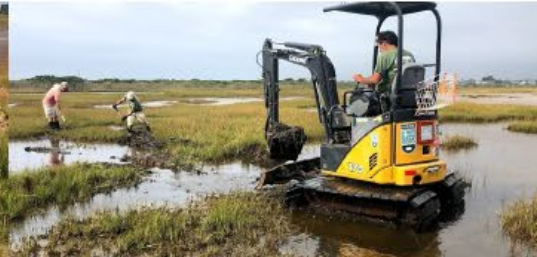
Creek excavation in fall of 2018 with low ground pressure excavator
