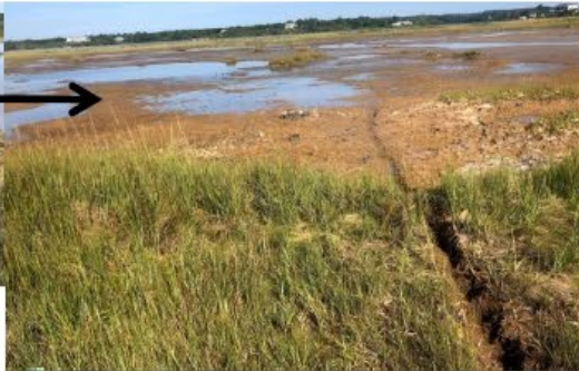
Runnel excavation by hand in summer of 2018
