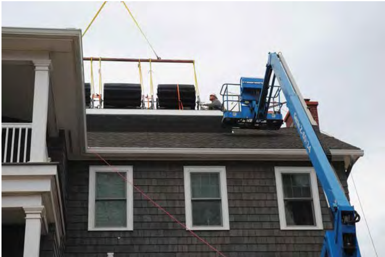
Workers install the first residential wind turbine in Ocean City on the Boardwalk at 14th Street. The new system should produce around 61,000 kilowatts of electricity each year—enough to power the condo for the summer. Photo courtesy of Ocean City Today.
