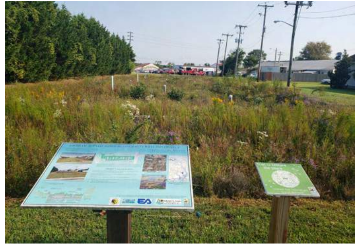
An old electrical transfer station was converted into a sand gravel wetland to collect and treat stormwater in a Berlin neighborhood prone to flooding. Photo by Roman Jesien.
