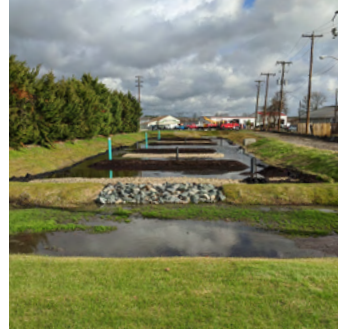
New sand-gravel wetland in Berlin designed to improve water quality.
