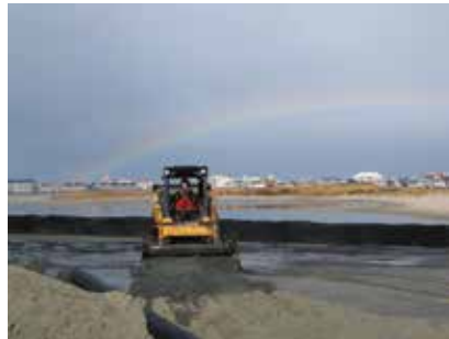
Huge pipes carry dredged sand and water from Sunset Marina to Skimmer Island, just north of the Rt 50 bridge. After the water decants, the sand is moved to renourish the depleted island. Within months of this effort horseshoe crabs and shorebirds make use of the new habitat. Photos by Dave Brinker and Carol Cain.
