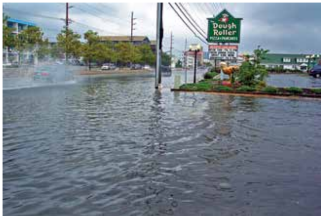
A summer thundershower floods Coastal Highway in Ocean City. Sitting only a few feet above sea level, Ocean City floods frequently, especially when rain events occur at high tide. Photo by Gail Blazer.
