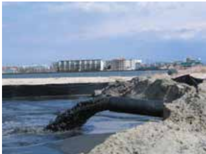
Huge pipes carry dredged sand and water from Sunset Marina to Skimmer Island, just north of the Rt 50 bridge. After the water decants, the sand is moved to renourish the depleted island. Within months of this effort horseshoe crabs and shorebirds make use of the new habitat. Photos by Dave Brinker and Carol Cain.
